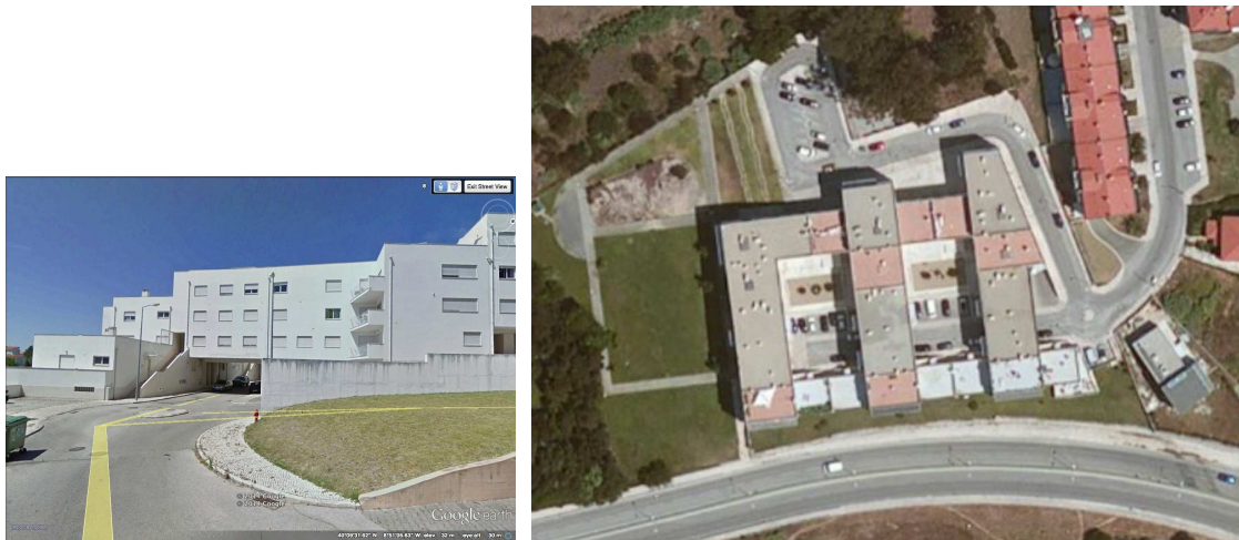
Figure 11. A two arch-building of private flats (private domain) over an urban road (public domain). (Source: Google Earth)
