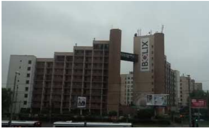
Photo. 3. Building with aboveground connector (photograph: www.panoramio.com ).
