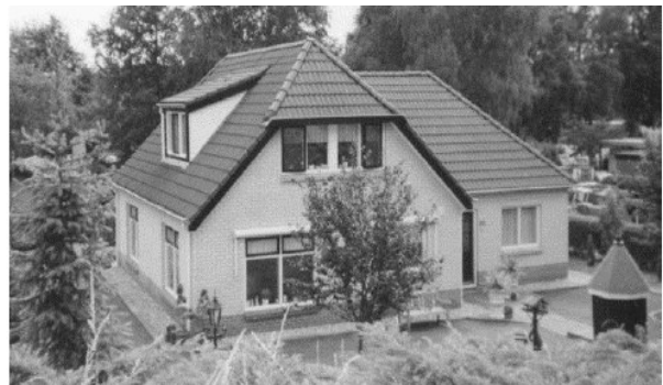
Figure 15 Photograph of the building.
