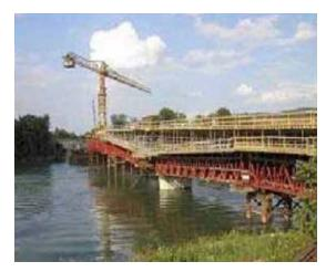
Bridge near Laufenburg collapsed due to altitude measurement difference of 0.54 m between Swiss and German side
