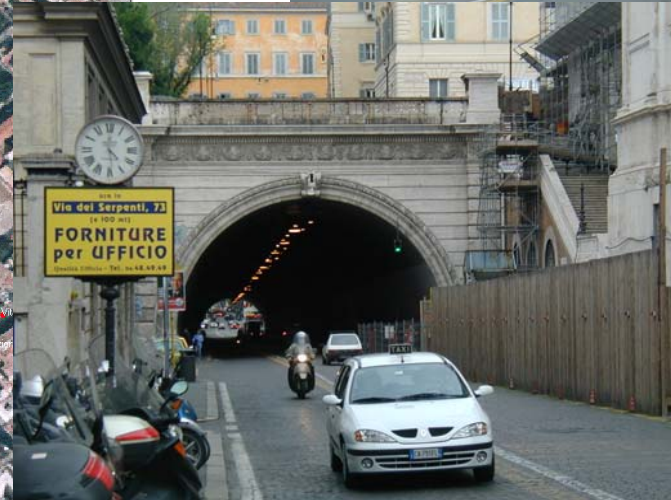
Tunnel Entrance (south-east)
