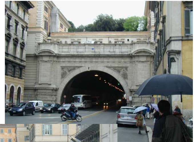
Tunnel Entrance (north-west)
