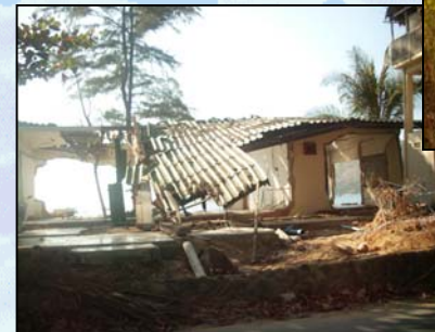
Nearby Tsunami damage
