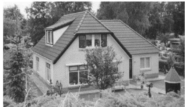
Figure 15 Photograph of the building.
