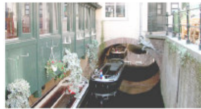
Figure 2 Multiple land use at one location: buildings on top of a canal.
