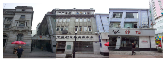
a Cross-road A b Connected building c Cross-road B Fig.24 Large range variance in raw images
