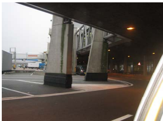
Fig. 11. Ring-road underpassing a pier at Schiphol Airport.
