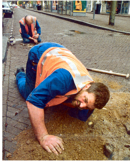
Figure 4.4: To avoid damage to cables, first digging by hand is necessary (De Volkskrant, (Dutch Newspaper), 6 July, 2000).
