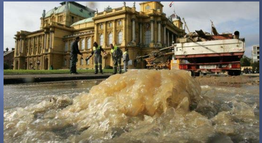
Water pipe perforated during survey activities for underground garage in Zagreb city centre – October 2010
