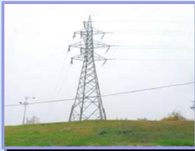
7. Power transmission tower and parcel below
