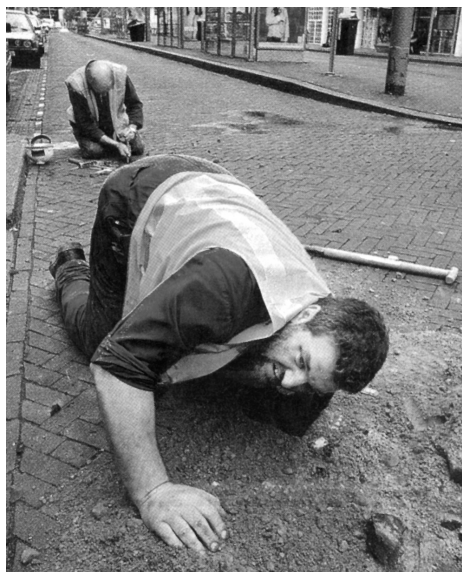
Figure 5: To avoid damage to cables, first digging by hand is necessary (De Volkskrant, (Dutch Newspaper), 6 Juli, 2000).
