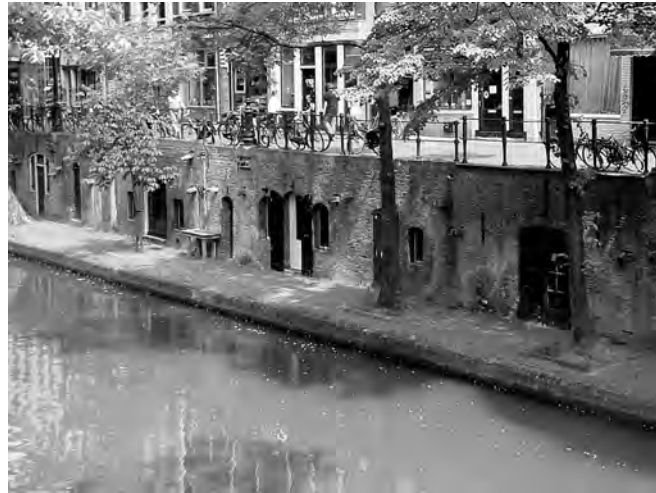
Figure 2.1: Cellars below roads in Utrecht.
