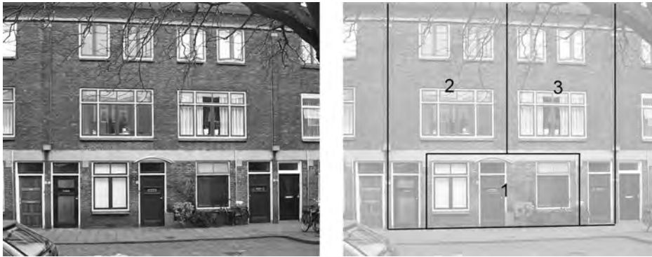
Figure 3.4: Apartment complex used in case study.
