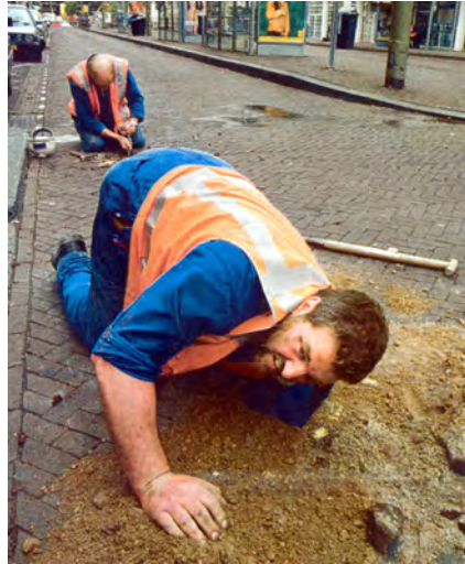
Figure 5.3: To avoid damage to cables, first digging by hand is necessary (Dutch Newspaper, July, 2000).
