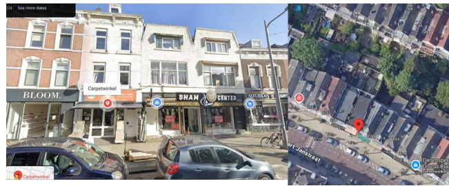
(a) Building location for Sample 1
