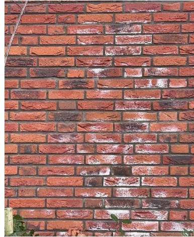
Figure 9 Early Onset of Efflorescence on a Newly Built Masonry Wall
