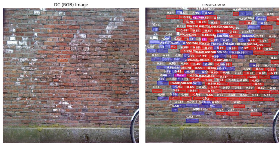
Figure 53 Efflorescence and damage predictions results with confidence scores (Epoch 60) (1) Original image. (2) Efflorescence and damage prediction.
