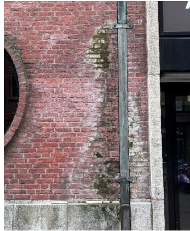
Figure 10 Efflorescence and Biological Growth Near a Drainpipe on a Masonry Wall
