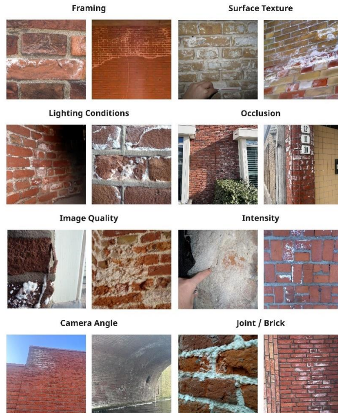
Figure 23 Visual examples of dataset diversity in efflorescence images. Variations in framing, surface texture, lighting, occlusion, image quality, intensity, camera angle, and efflorescence location
