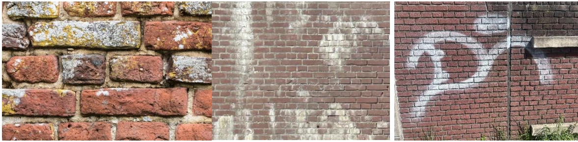
Figure 5 Examples of surface phenomena visually similar to efflorescence on Dutch masonry: (left) biological growth (lichens/mold) on a historic brick façade, (middle) encrustation deposits on a quay wall in Amsterdam, and (right) graffiti on a masonry wall in Delft
