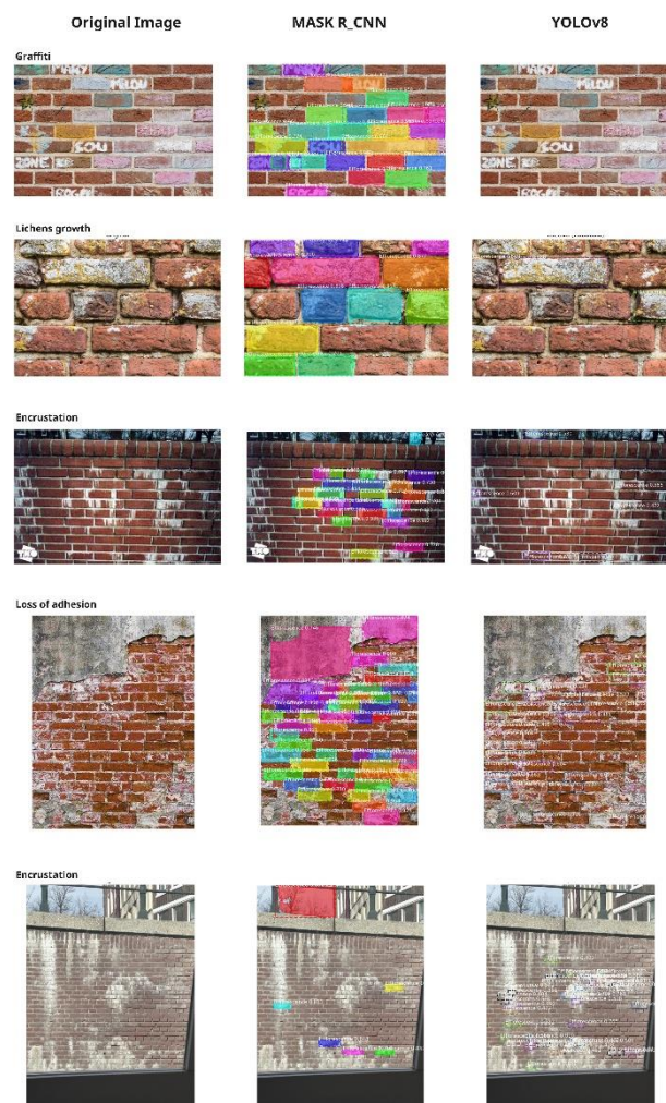
Figure 36 Comparison of detection results of non-efflorescence damages.
