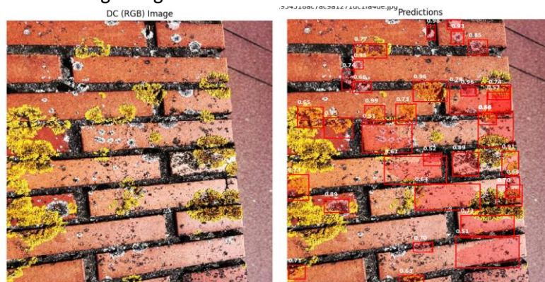
Figure 47 Efflorescence and Lichens predictions results with confidence scores (Epoch 60) (1) Original Lichens image. (2) Lichens prediction
